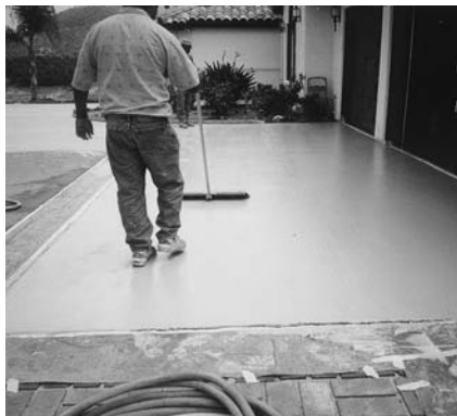
Broom immediately behind the metal squeegee to leave the desired texture.
