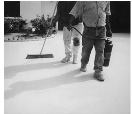
7. Apply Sealcoat 1000 using a pump up sprayer and a soft flagtip broom.
