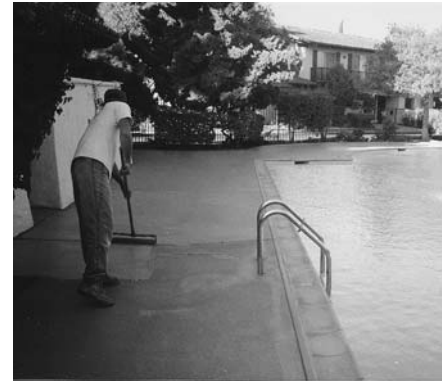
6. Apply Concrete Colorcoat using a paint roller.
