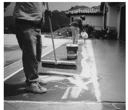
3. Before the first row of material runs out pour another row on top of it and if necessary spray more water where needed.
