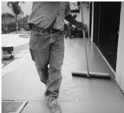
2. Spread the Fine Broom Finish material to a thin even coat next to the starting edge using a metal squeegee and broom to the desired finish.
