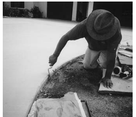
Scrape or brush the vertical edges where the material drips over the sides.
