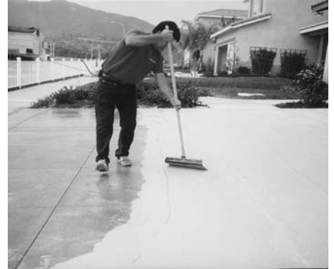
Apply a Squeegee/Bond Coat using a 24" Metal Squeegee.
