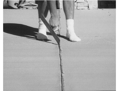
4. Scrape out any material that got in the joints using a trowel or scraper before it dries too hard.
