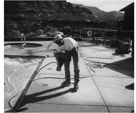
Spray the Spray Texture Mix over the surface using hopper gun spray unit.
