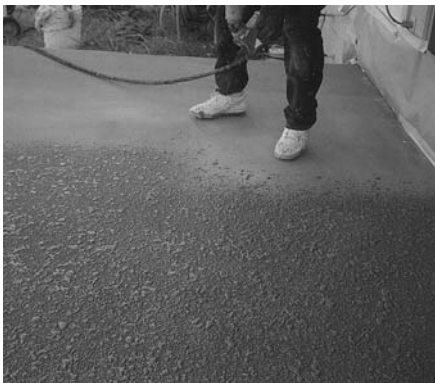
1. Spray the Spray Texture Mix at a 75-80% coverage rate to achieve an even textured profile.
