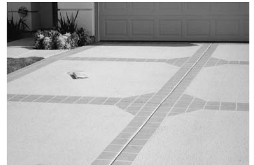
Decorative borders or stencil patterns can be applied to enhance the appearance of the Spray Texture Finish.
