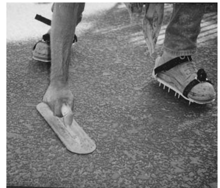
3. While wearing spiked shoes knock the spray texture down flat before it dries using a trowel.
