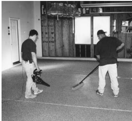
Scrape surface and blow to remove loose flakes
