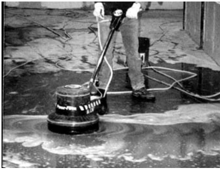
Detergent scrub, acid wash, neutralize
