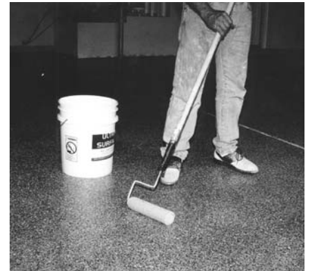
Apply second coat of SB Urethane
