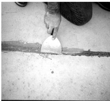
Fill cracks w/ Sealcoat 500 epoxy & sand
