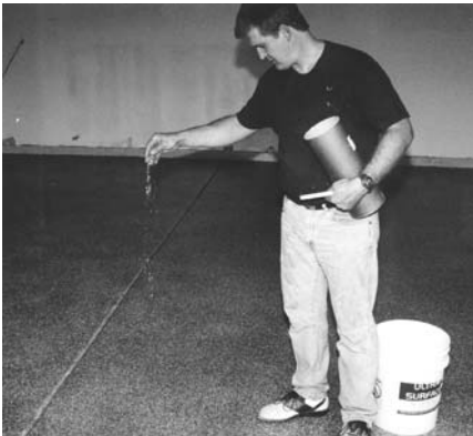
Sprinkle flakes into urethane if needed to even look
