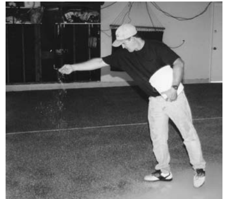
Sprinkle flakes in thin areas or next to edges
