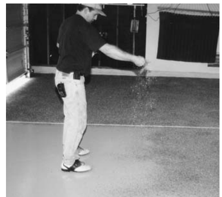
Sprinkle by hand for light to medium coverage
