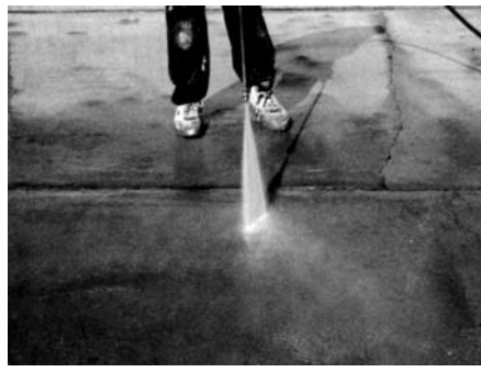
Pressure wash surface to clean and rinse
