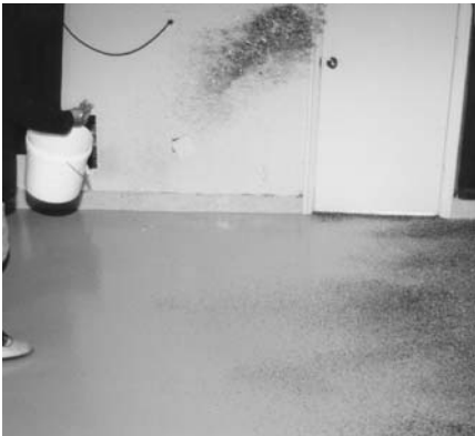
Method1: Throw flakes up in the air by hand
