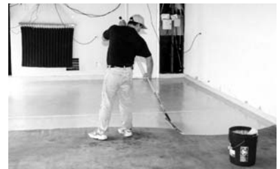
Apply Epoxy 200 with metal squeegee
