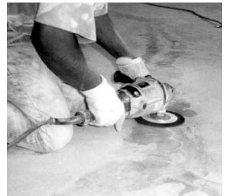
Grind epoxy over crack, smooth w/ surface
