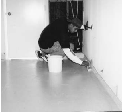
Apply WB Epoxy or SB or HP Urethane to edges
