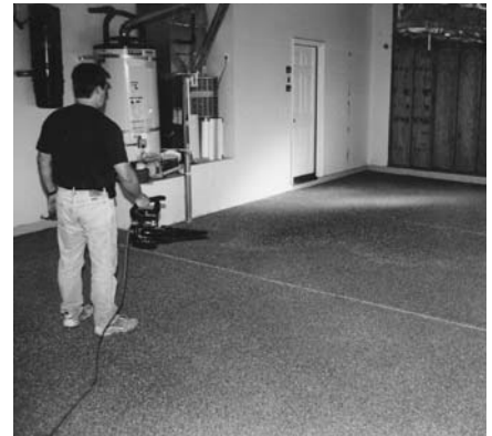
Blow loose flakes to thin areas only if needed
