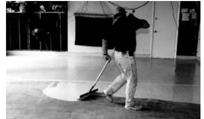
Apply a Squeegee bond coat if needed
