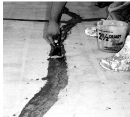
Scrape excess epoxy, leave little above crack
