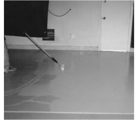
Spread thin w/ 3/8" nap paint roller
