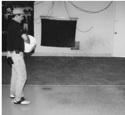
Cover epoxy or urethane completely w/ flakes
