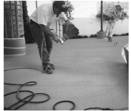
15. Apply desired finish
