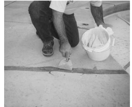
3. Fill with Epoxy 500 sand mix.
