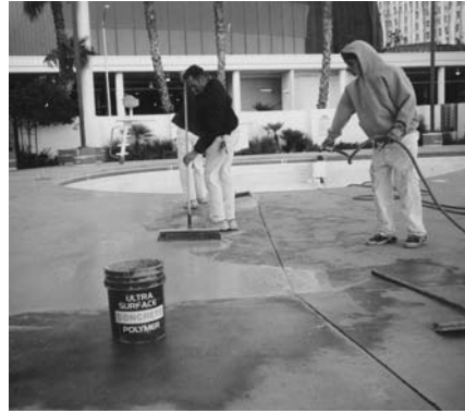
14. Apply a squeegee coat over entire surface
