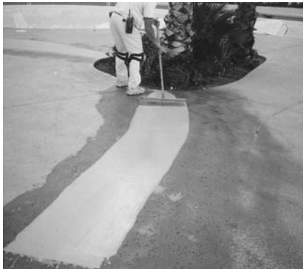
10. Pull the material to a pile
