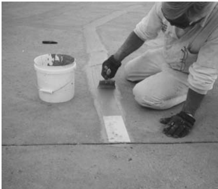
7. Apply Elastomeric Basecoat over fabric.
