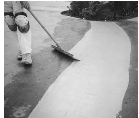
12. Scrap edges and feather to zero
