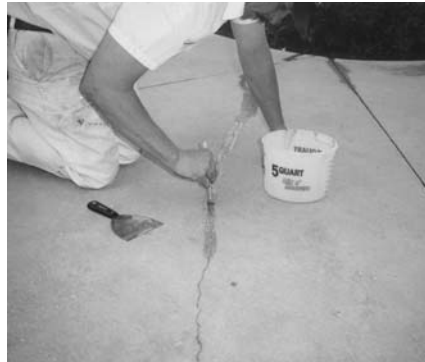
2. Prime with Epoxy 500.
