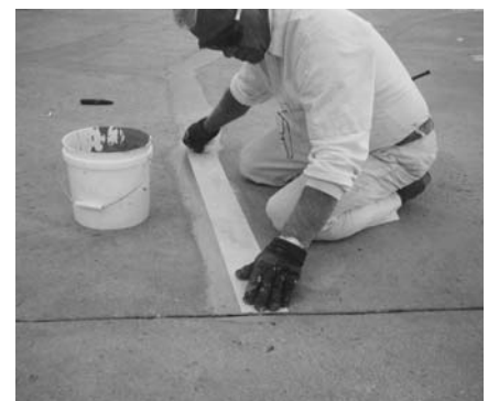
6. Lay crack repair fabric over E. Basecoat.
