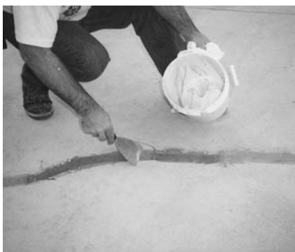
4. Scrape up excess sand mix.
