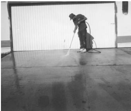
1. Pressure wash cracks.
