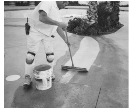
9. Spread patching mix over crack repair.
