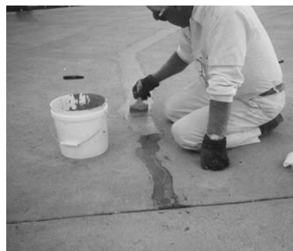
5. Apply Elastomeric Basecoat over S-500.
