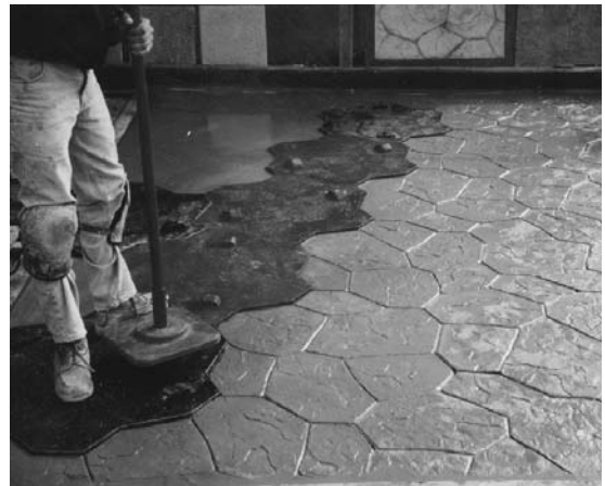
1/4" stamped concrete finish
