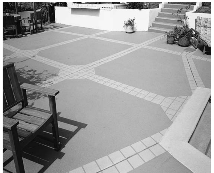
Trowel Knockdown Texture With Tile Border Design.
