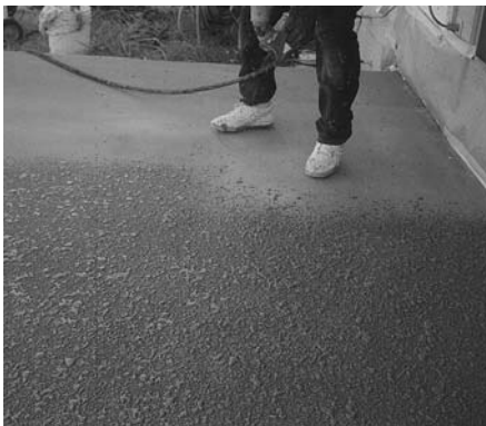
1. Spray the Trowel Knockdown Mix at a 75-80% coverage rate to achieve an even textured profile.
