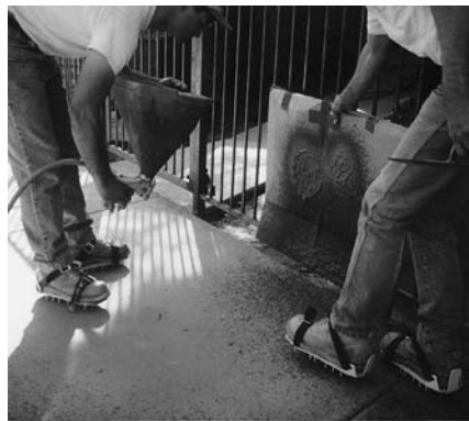
2. Mask off surrounding areas to prevent over spray or use a cardboard shield next to the edges.
