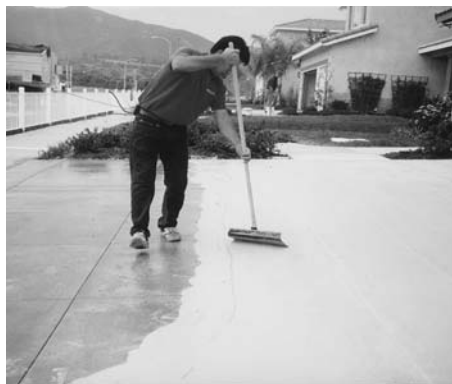
Apply a Squeegee/Bond Coat using a 24" Metal Squeegee.
