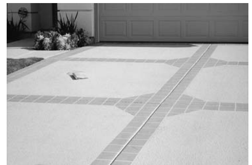
Decorative borders or stencil patterns can be applied to enhance the appearance of the Trowel Knockdown Finish.
