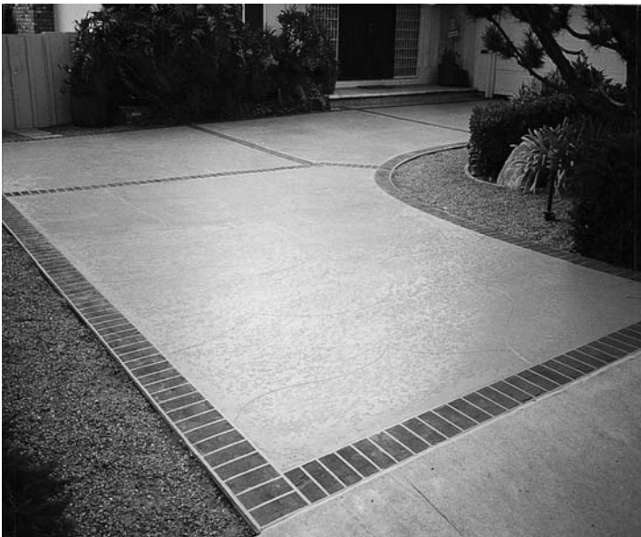
Trowel Knockdown Texture With Brick Border Design.
